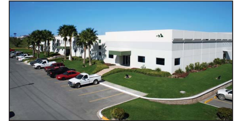
Del Norte Facility - Reynosa, Tamaulipas, Mexico
